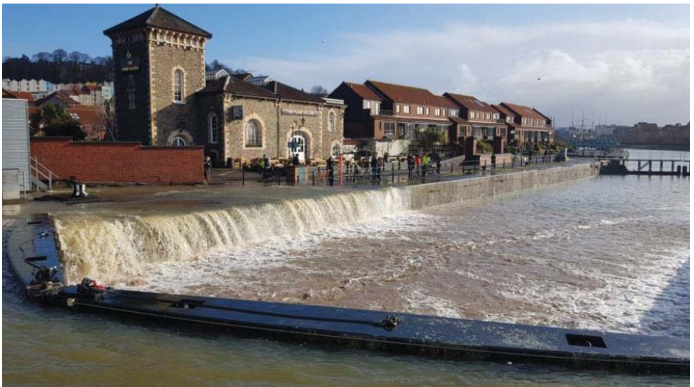
Figure 37: Overtopping at Junction Lock during March 2020 tidal surge
