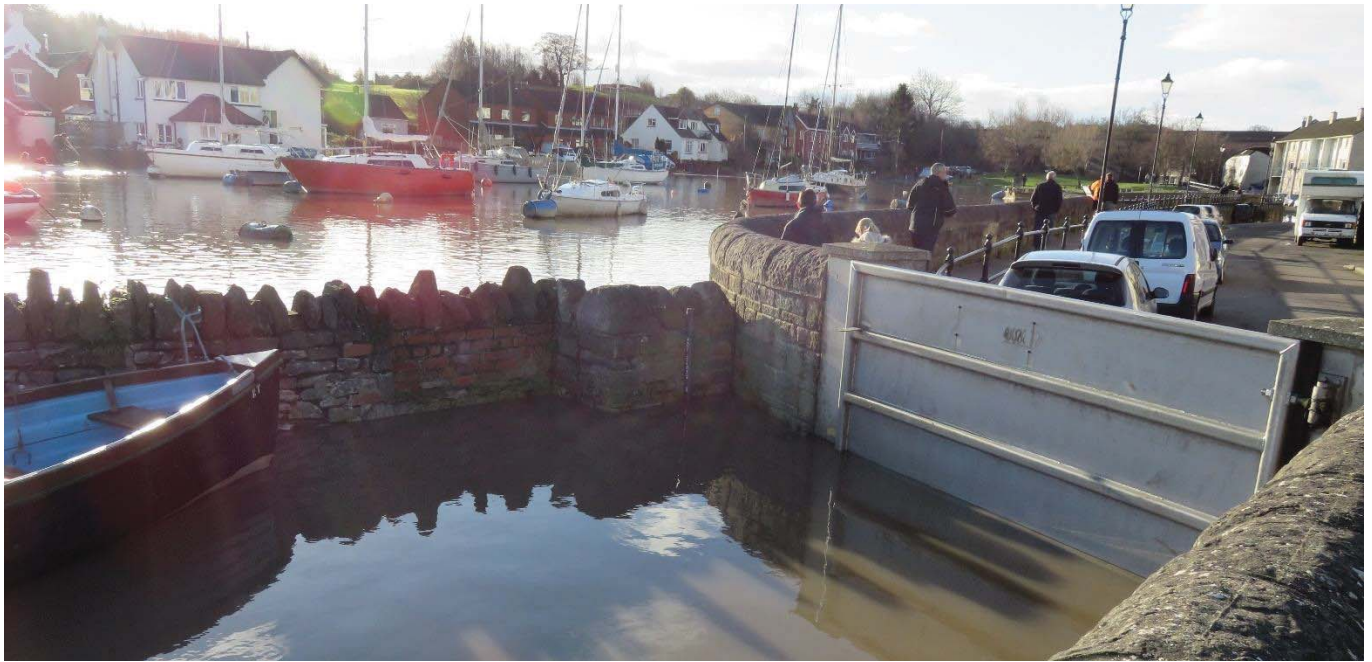
Figure 25: Existing flood defences in operation at Pill
