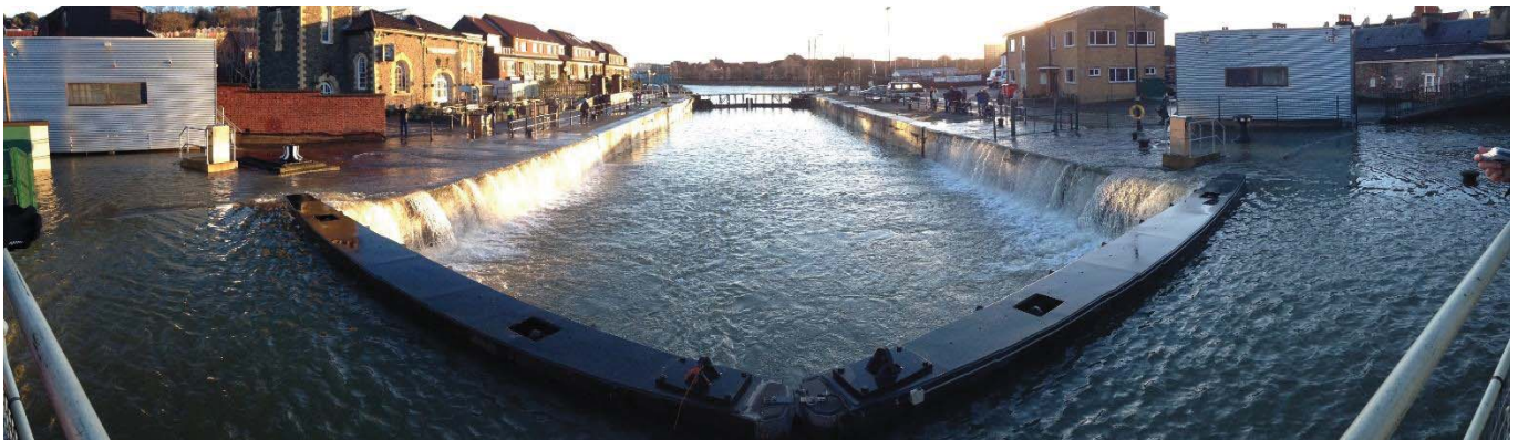
Figure 1: January 2014 tidal surge inundating the A4 Portway in the Avon Gorge (top), Cattlemarket Road (left) and Clarence Road (right), and outflanking tidal flood gates at Junction Lock into the Floating Harbour (bottom).
