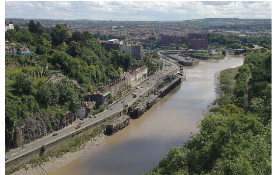
Figure 8 View of Entrance Lock from downstream
