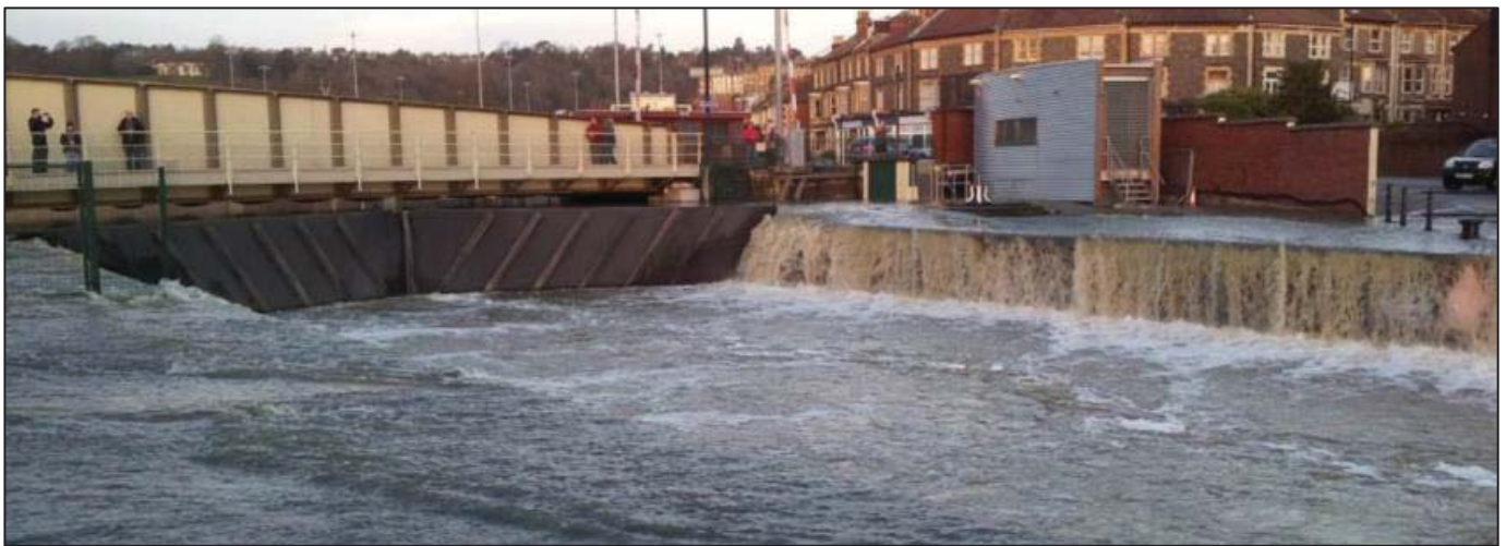
Figure 19: Water shown overtopping the Junction Lock stop gates into the Floating Harbour
